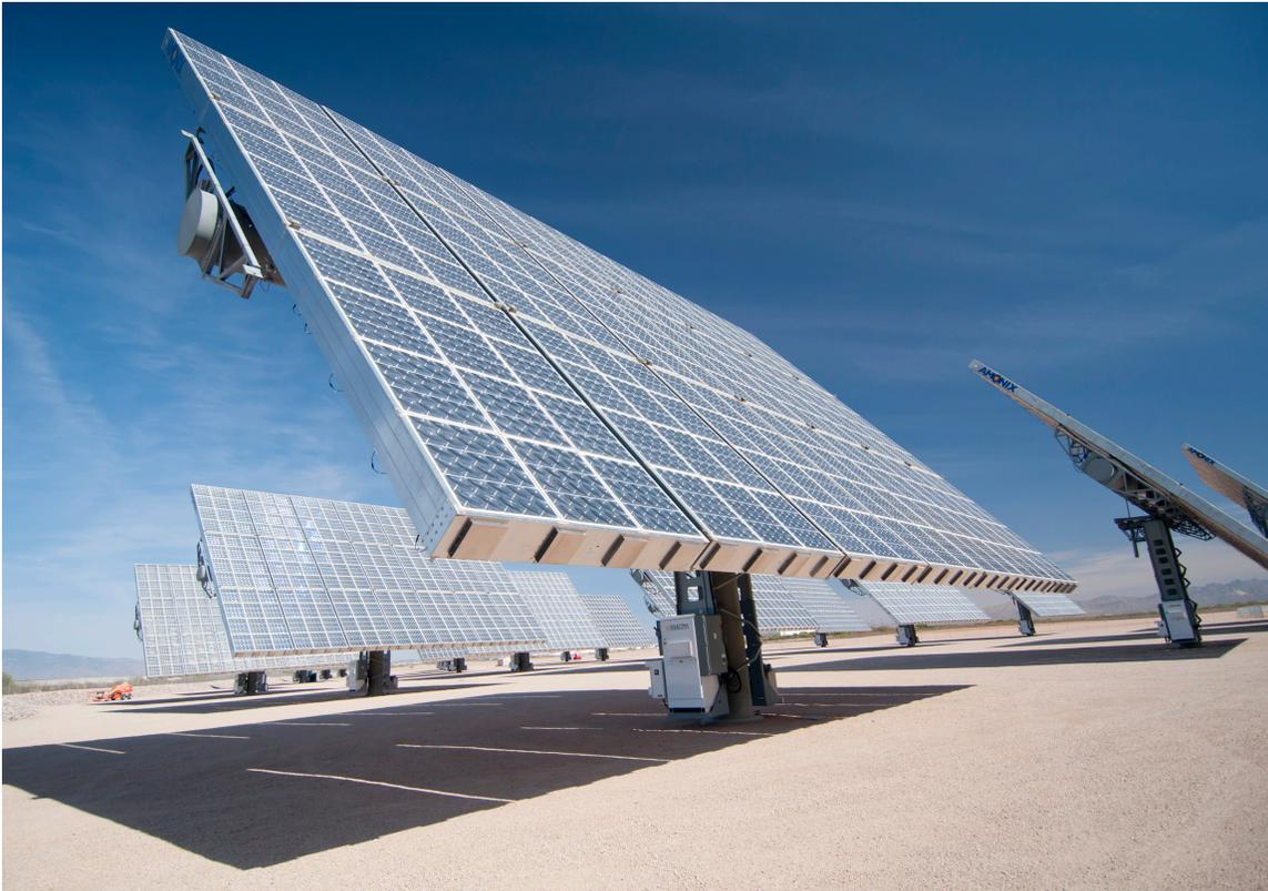
Fig. 2. This is an image of the Universal Module from Arzon Solar LLC in a utility scale generating facility. This is a concentrator photovoltaic system, implementing lenses that focus light onto small multi-junction solar cells. Note the large size and height of each module, as opposed to single junction solar cells that are much smaller. Also, compare the blue sky to Fig. 3.
