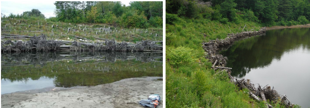
Figure 6. Two views of the rootball revetment at Stop 4 in Farmington Falls, 2014 (left) and 2017 (right). Initially, it was easier to see the shorter trunks, but as vegetation has established itself (right), only the rootwads at water level are easily visible.
