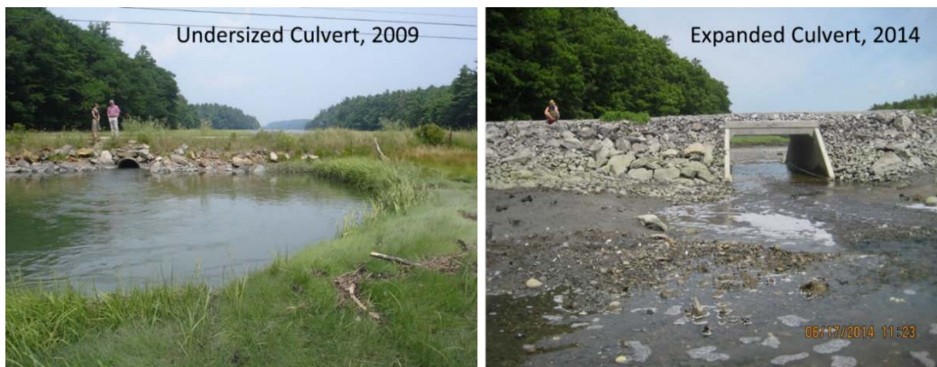
Figure 7. Culvert at northern end of Long Marsh, prior to and after the 2014 restoration.
