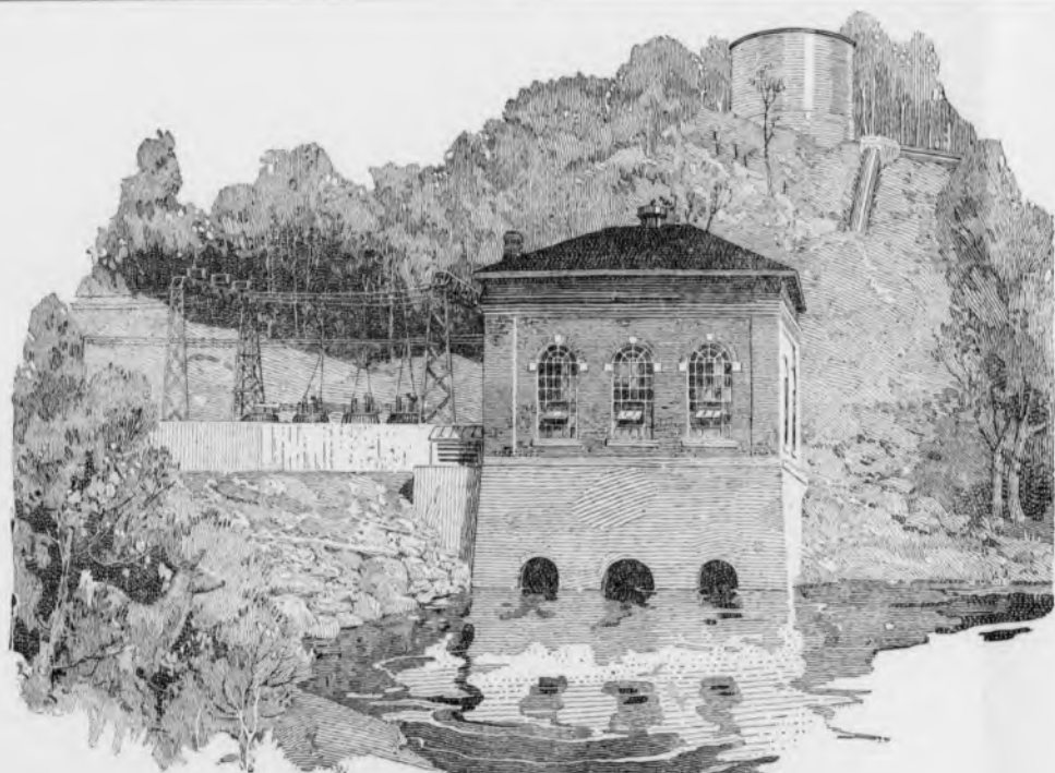
In an isolated region, almost inaccessible in winter, this 6500 h.p. hydro-electric plant located on the Deerfield River in New England, starts, protects, and stops itself.
