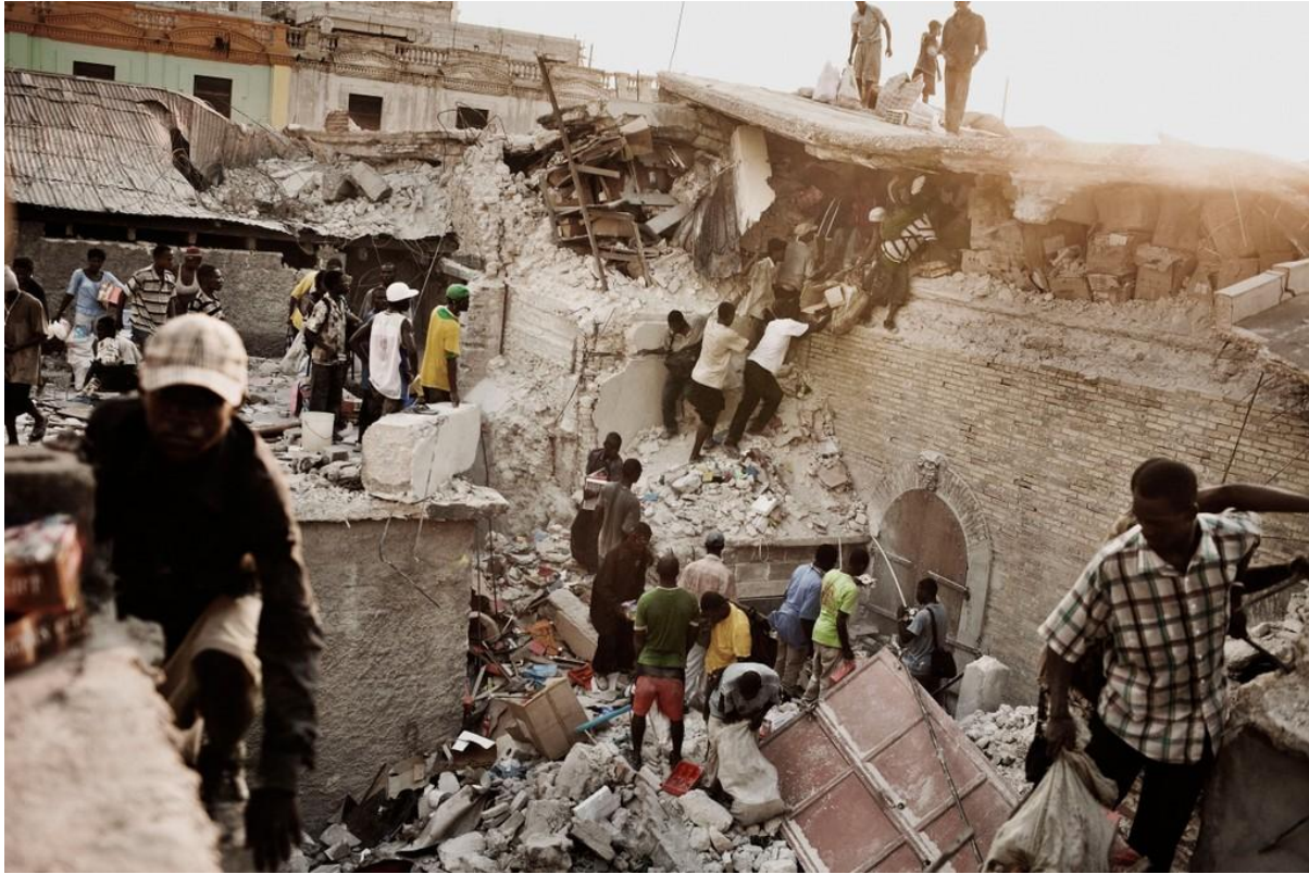
Fig. 13. Community members saving valuable resources from a collapsed earthquake in Port-au-Prince seven days after the earthquake; Moises Saman. HAITI. Port-au-Prince. January 19, 2010. Haitian Try to Salvage Any Valuables from a Destroyed Warehouse in Downtown Port-au-Prince in the Aftermath of January 12th's Earthquake. JSTOR, https://jstor.org/stable/community.18995905 . Accessed 27 Mar. 2023.
