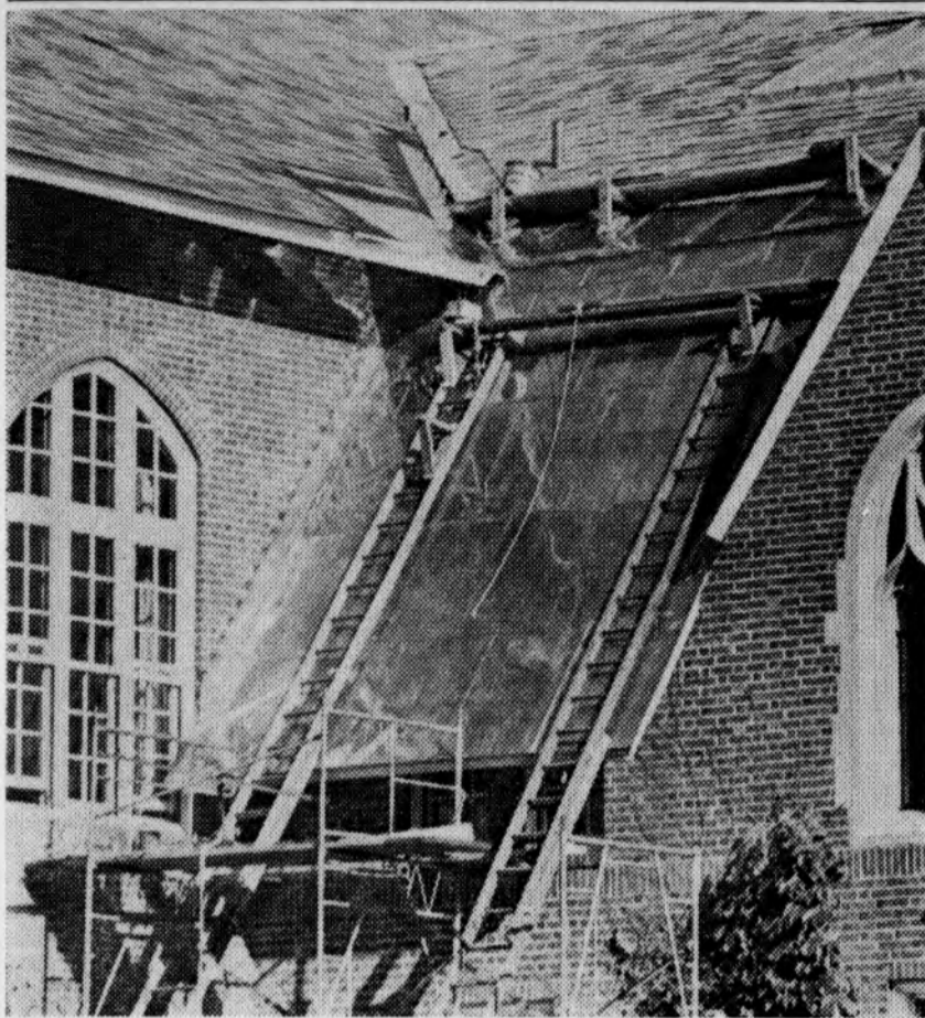
Repairs to the Gym. It Won't Help!
