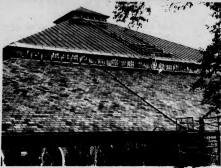
Ongoing replacement of broken panes on the top of The Cage
