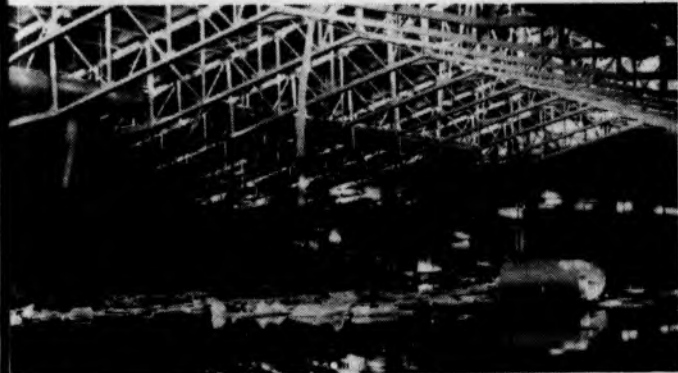
Parts of the roof of the new gym must be re-fitted.
