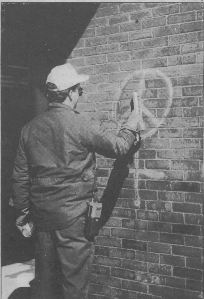
Maintenance employee removing graffiti from the wall of the library. File Photo.
